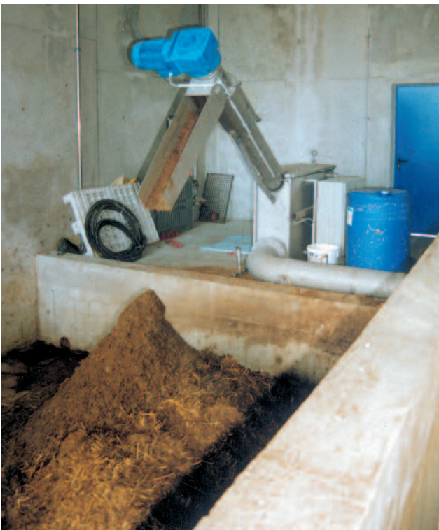
Slaughterhouse Ingolstadt / Germany Top: ROTAMAT® Micro Strainer Ro 9, HUBER Dissolved Air Flotation Plant HDF-3 with chemical treatment, throughput: 30 m³/h Left: Truck washing with ROTAMAT® Micro Strainer Ro 9 in tank, final DS > 35 %
