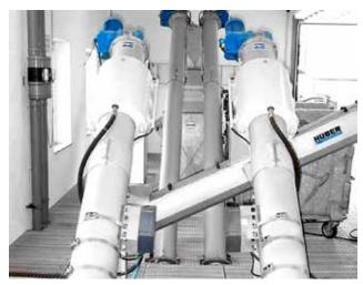
Underground, redundant HUBER Complete Plant ROTAMAT® Ro5.
