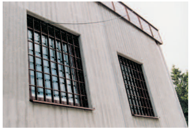
Window protection grilles
