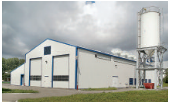
Turn-key HUBER dryer with two parallel trains and product silo
