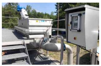
Process wastewater screening for textile fibre separation.
