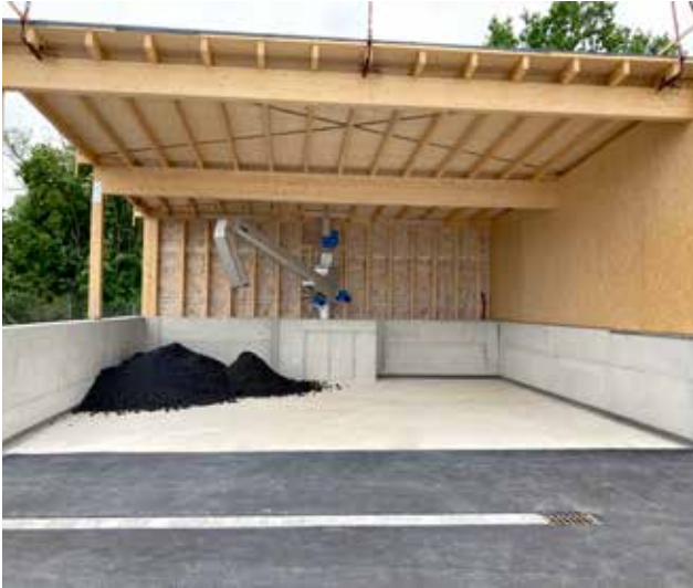
Sludge discharge through the Ro8 TC to a free area...
