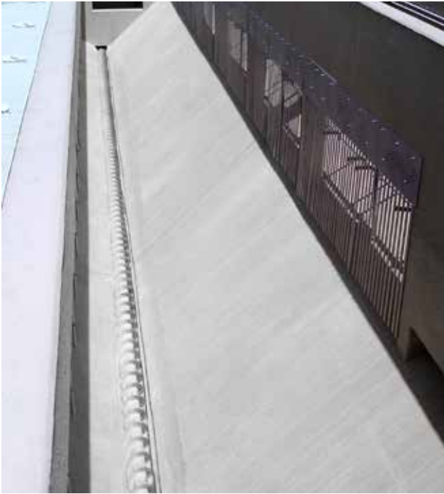
HUBER Trough Screw Conveyor Ro8 T as grit removal screw in a longitudinal grit trap.
