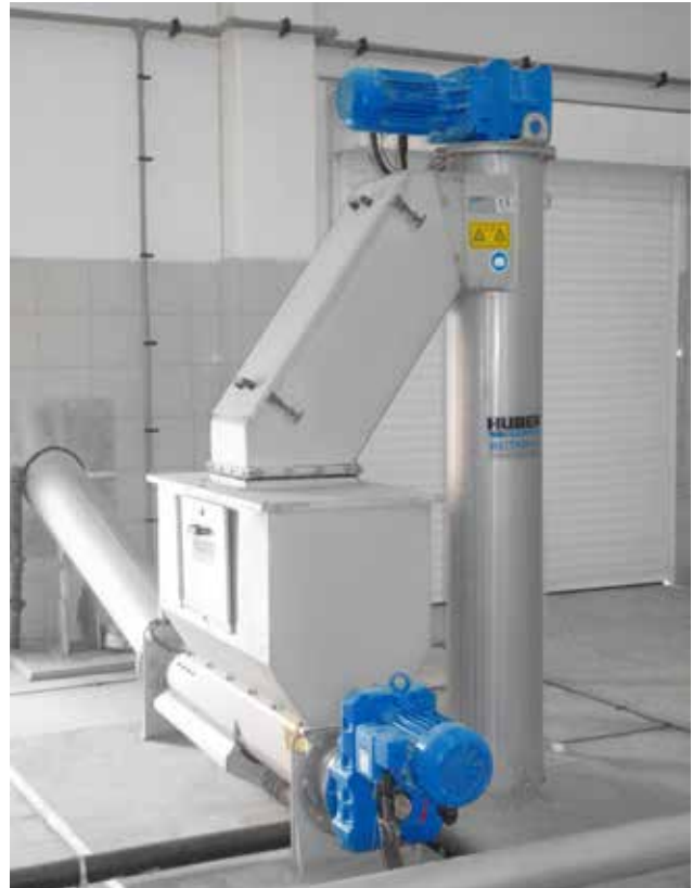
Vertical installation of a HUBER Screw Conveyor Ro8 discharging screenings into a HUBER Wash Press WAP®.
