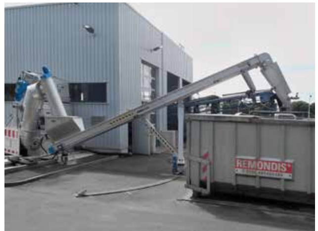
Rotating Screenings Distribution Screw Ro8 TC.
