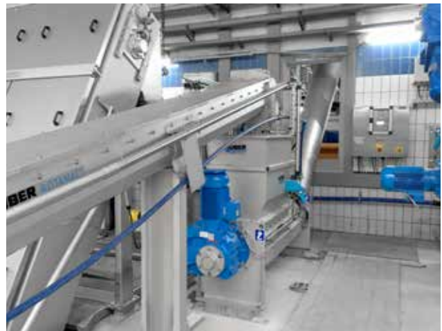
Conveyor solution for mechanical pre-treatment of unpressed screenings.
