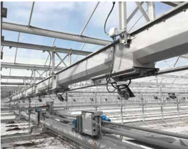
Distribution conveyor to supply sludge to a HUBER Sludge Turner SOLSTICE®. 55 m conveyor length, 16 discharge points.
