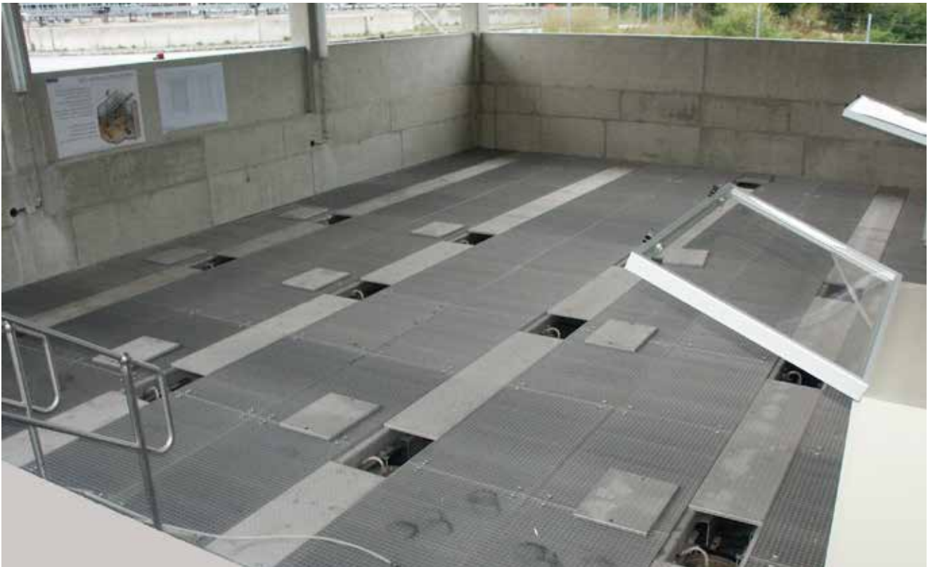
HUBER Active Carbon Filter CONTIFLOW® GAK (tank design).
