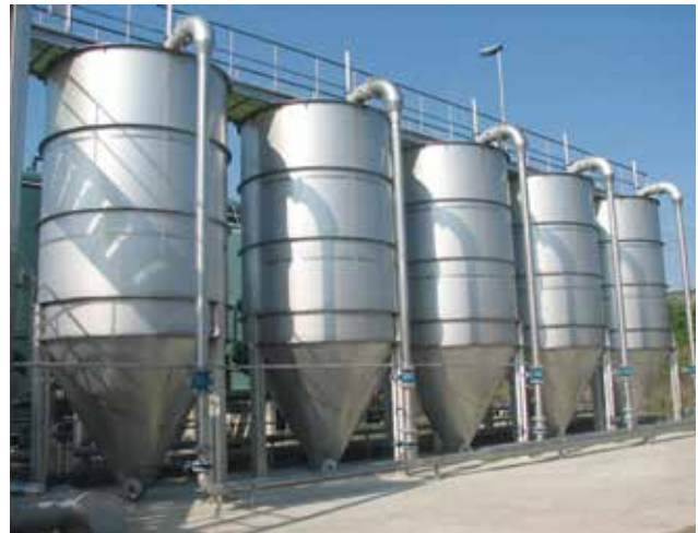
HUBER Sandfilter CONTIFLOW® 72, Montebello, Italy.
