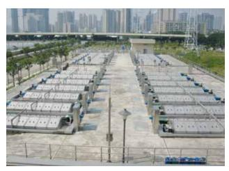
28 HUBER Disc Filter RoDisc® units with 24 discs each treating about 8.5 m³ wastewater per second.
