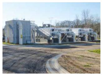
4 HUBER Disc Filter RoDisc® with 18 discs in stainless steel container.
